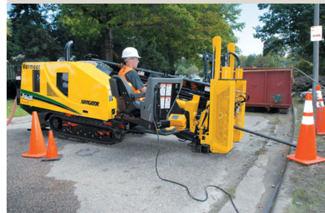
Directional drilling minimizes impact (right)
